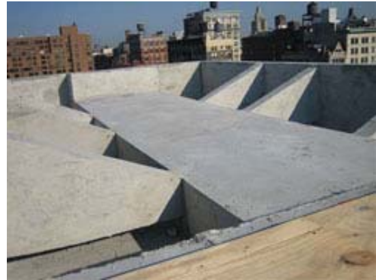
Figure 6 –Penthouse Roof Structure
